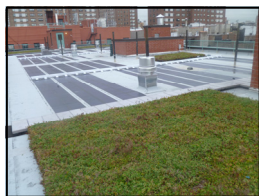
Combination solar and green roof at Kurt & Leah Schneider Apartments.
