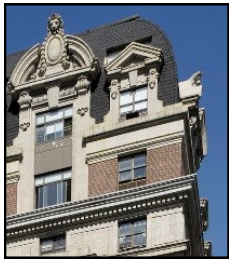
Facade detail at the Marseilles
